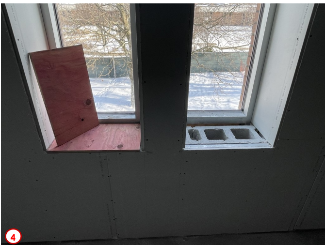
Photo #3 highlights the progress of some of the finer finish work happening as far as the installation of the wallboard is concerned. Here the soffit that will serve as the transition from the suspended ceiling to the hard ceiling near the window has received its board and will be finished after.
