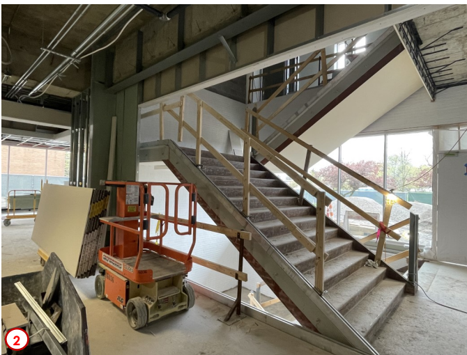
Photo #3 highlights the progress of the work in the library near the area of the new huddle rooms along the south side. Here you can see the wallboard in place and now taped and mudded. Once sanding is complete these walls will be painted.
