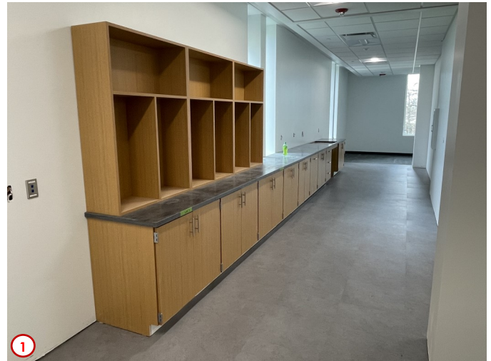
Photo #1 was taken near the kitchenette in the new H/SS Division Office Suite. Here you can see all the new cabinetry in place along with the new countertops. The closer end is where all the adjustable shelving will be placed that will serve a mail slots for the faculty, and then at the far end will be where the sink, microwave, and refrigerator will be installed.
