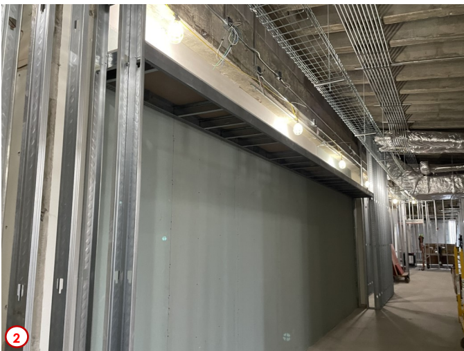
Photo #3 was taken in the future H/SS Office Suite entry lobby. Here you can see that the wallboard continues to be installed. Now in addition the walls are receiving batt insulation that will help deter sound transmission and assist in achieving a quieter office area for faculty.
