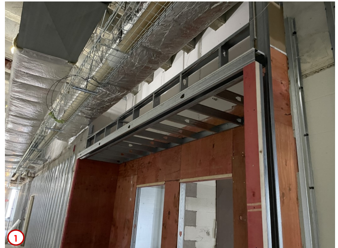
Photo #1 shows some of the typical detailed framing that is happening at each of the classroom entry ways. This new constructed bulkhead will receive wallboard at a later time to help finish it out. It is areas like this which will receive special finishes that will help with wayfinding, and add character and help provide a nicer overall environment throughout the building helping it to have a warmer and pleasant feel as opposed the colder more sterile feel that used to exist in the building.
