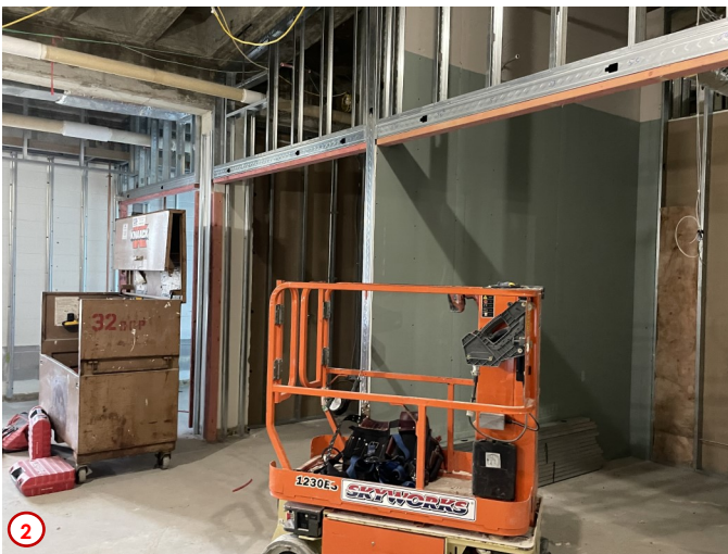
Photo #3 shows the wall near the now open west stair tower and the metal furring strips now installed. Wallboard will be hung on these strips, and so to accommodate this new finish the old door frames were removed so new compatible versions can be installed.
