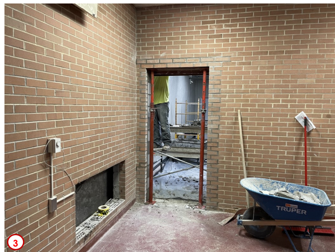
Photo #2 shows the progress of tooting in the concrete block so that the new door and frame for the new Janitor's Closet can be installed later. The irony of this photo is that the level of the scaffolding is where the new floor will be later (once erected) for the new closet, however you won't be able to see it from inside the existing mechanical room as it will be covered and held in place by perimeter walls made of concrete block.
