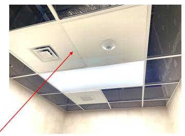
The top-right photo shows the ceiling in the new unisex restroom nearly complete. Now that all the mechanical and electrical items have been installed the remainder of the ceiling tile can be installed.
