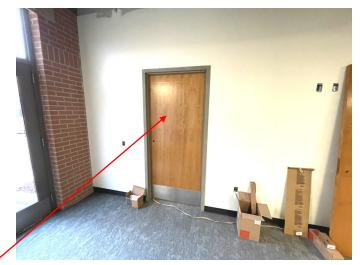
The top-right photo shows the new wood door in place for the unisex restroom. The door handle and lockset still needs to be installed. The same situation goes for the private room next door.
