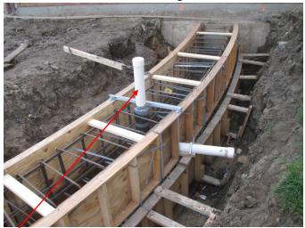
The top-left photo highlights not only the completed formwork for the addition foundation, but some of the infrastructure that needed to be completed prior to placing the concrete. Here you can see one of two stub-outs that will connect the roof drains to the storm sewers.
