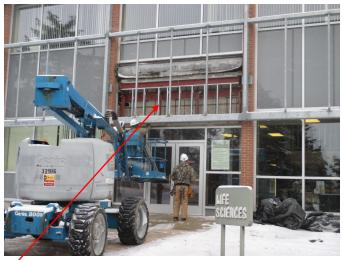
The top-left photo shows some of the work earlier this week above the south entrance of the existing building. You can some new lightgauge metal framing has been added. Next the contractor will install some wood sheathing and then eventually some corrugated metal panels to match the north side of the building and addition.
