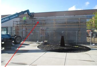
The top-left photo highlights the progress of the construction of the cmu wall that forms the north side of the new addition. This wall be clad in metal panels on the exterior similar to those on the CTC.
