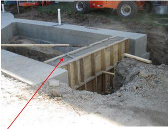
The top-left photo shows another portion of the foundation system being completed. Here the part of the foundation that forms the frost-proof stoop for the new addition entry has been formed and the concrete placed.
