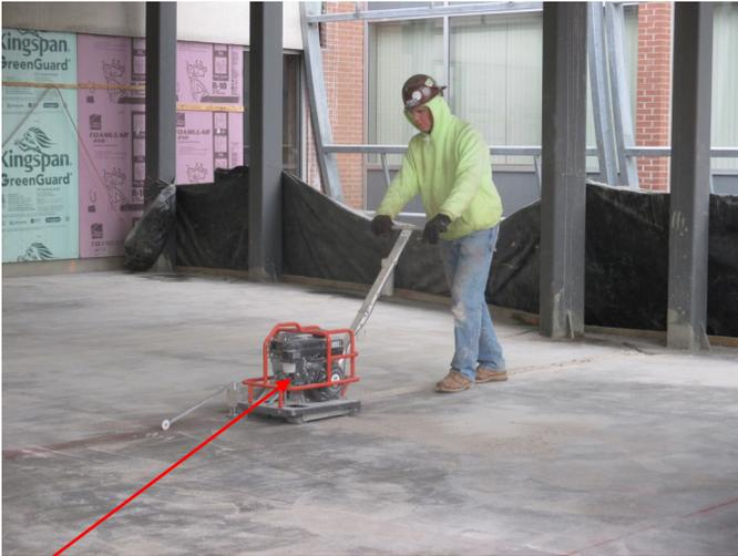
The top-left photo shows one of the contractors cutting the control joints in the floor slab. This joint will help to keep cracks in the future from telegraphing through the slab.
