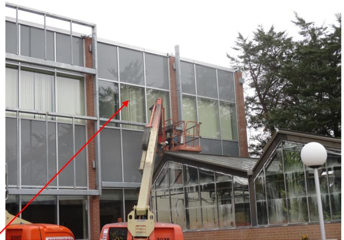
The top-right photo highlights the installation of the last few bays of support steel on the south face of the building. The installation of the steel in this area will take a little longer as it is more difficult due to working around the greenhouse and connecting corridor.
