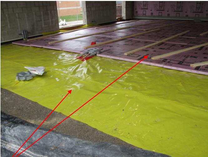
The top-left photo highlights the preparation for the installation of the concrete floor slab of the addition. Here you can see the under slab vapor barrier and rigid insulation being placed.
