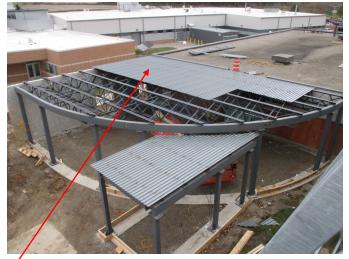
The top-left photo shows the progress of the installation of the metal decking for the addition roof. Once completed a thin layer of concrete will be placed on top to help create rigidity in the addition.
