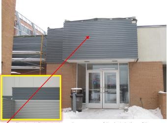
The top-left photo shows the progress of the installation of the new corrugated metal panels that are being installed over the existing precast panels on the north wing of the building. These panels match what is already installed on the neighboring CTC Building as shown in the smaller picture in the corner.
