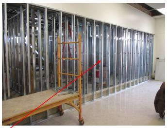
The top-left photo highlights the new double-stud wall that will separate the addition from the existing building. This wall will be filled with insulation in order to acoustically protect the end classroom from noise being generated in the addition.
