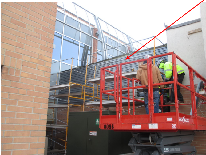
The bottom-left photo shows the beginning of the installation of the new corrugated metal panels that will be installed over the top of the existing precast concrete panels. This will also help to tie the Life Sciences Building and CTC together from an appearance standpoint.
