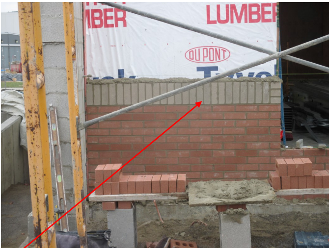
The top-left photo shows the beginning of the installation of the new brick veneer on the addition. Unlike the rest of the existing building the addition will have a brick accent band that will help it relate to the CTC better aesthetically.
