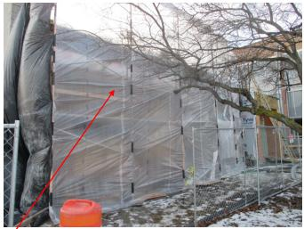
The top-left photo highlights the construction of some temporary tenting that will be used so the masons can finish the brick veneer on the exterior of the addition. This area is heated so as to allow the mortar to set up properly and be workable for the masons.
