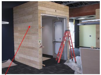
The top-left photo shows the progress of the installation of the Kieri brand board. This board is a sustainable product made out of sorghum straw. After installation it will be sealed to help protect it. When you look at the board up close it has an almost plant or animal cell feel to it which we thought was fitting for a science building.
