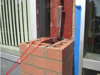
The top-left photo shows a detail of the new brick ribs that are going up between the existing sections of curtain wall systems. Here you can see a new stirrup-shaped horizontal tie hooked into an existing slotted anchor connected to the building frame. This tie anchors the brick piers to the building, and the slotted anchor allows for the materials to expand and contract at different rates to avoid cracking.
