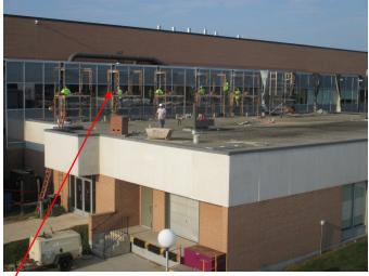
The top-left photo shows the masons constructing the new brick ribs above the north classrooms. Once the brick ribs are completed a partial roof replacement will be completed as part of the project.
