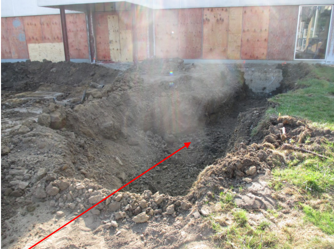
The top-left photo shows the excavation for the footings for the addition. Last week the top soil was stripped in this area. Once all the trenches are dug the contractor will place the forms.
