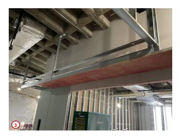
Photo #4 shows some of the need supports for future countertops, shelving systems, etc. now in place. With all of this infrastructure in place the wallboard can be finished.
