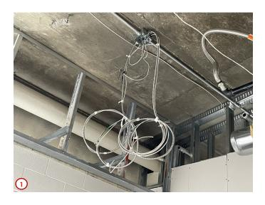
Photo #1 features one of the many instances where the wires have been pulled and whips ready to connect to the future lights in the ceiling in the H/SS Division Office Suite.
