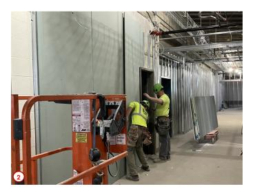
Photo #3 highlights more of the progress on the miscellaneous framing on the second floor. Shown in this photo is one of the many bulkheads that are being constructed in the area that will serve as transitions between varying types of ceiling systems.
