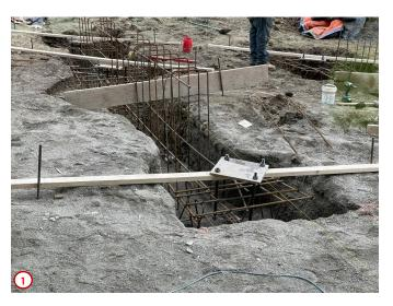
Photo #1 was taken outside the future east entrance on the first floor, and shows the trench excavated for the foundation system for the new canopy that will be installed in this area. You can also see the steel reinforcing bars and location for the anchor bolts will allow the structural steel to anchor to the foundation.
