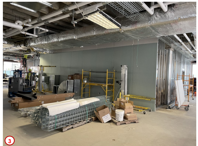
Photo #4 shows the area of the future addition to the southeast corner of the building. Looking at the photo you can see the wire-mesh reinforcing in place and the dowel rods that will help support the floor slab and connect it to the existing slab respectively. Next week this concrete will be placed along with the foundations for the screen enclosure, west entrance canopy, and the new door stop at the base of the west stair tower.
