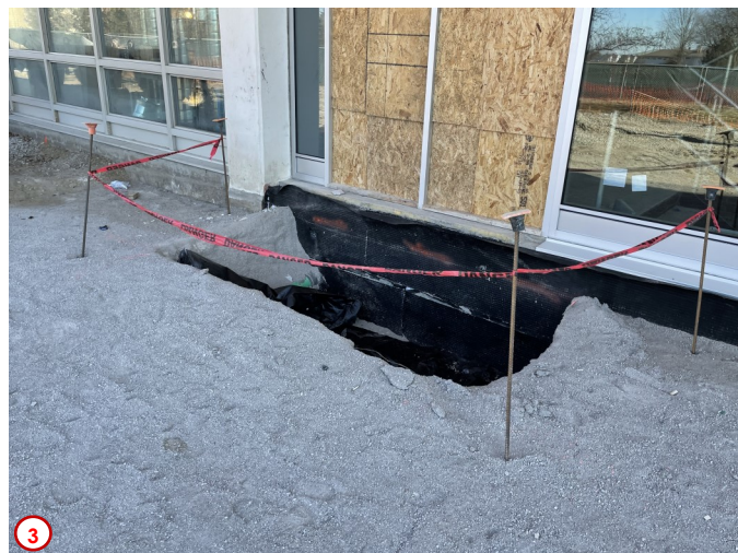
Photo #2 shows the foundations for the future entrance canopy on the east side of the building. You can also see the connecting reinforcing steel that will help connect the future partial height seating walls sticking up out of the concrete. Additionally, the anchor bolts (wrapped in the red tape) are in and these will help anchor the steel support columns for the canopy.
