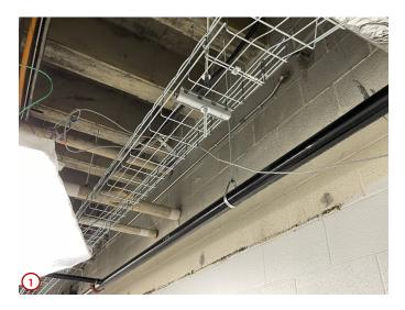
Like the 2nd and 1st floors the basement is now having a lot of its above ceiling infrastructure being installed. For example, in Photo #1 one can see not only the aforementioned fire sprinkler main trunk lines now in place, but now next to the cable tray is in that will hold all of the new data cabling that will feed all the classrooms, offices, etc. in the area with network connections stemming from the main server in the southwest corner of the basement.
