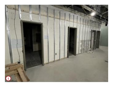
Photo #1 shows some new door frames that were installed this past week. Here there were four different existing door frame scenarios that had to be dealt with, so in order to make everything work correctly and look cohesive new frames were installed that will properly receive the new wallboard planned for this area.
