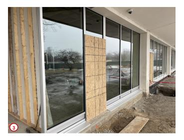
Photo #4 shows the now cured concrete floor slab for the southeast addition. With both floor slabs ready to receive the new curtain wall systems. When all these are installed the total perimeter of the first floor will then be complete and weathertight which then aids with the interiors of the building being able to be installed.
