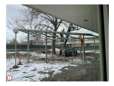
Photo #1 was taken earlier in the week and shows the contractors erecting the steel structure for the new east entrance canopy. At ground level you can see the reinforcing stirrup bars coming up out of the footing that will both support the concrete seat wall that will be placed and also structurally reinforce it. The concrete for the seat wall will be placed when the weather improves.
