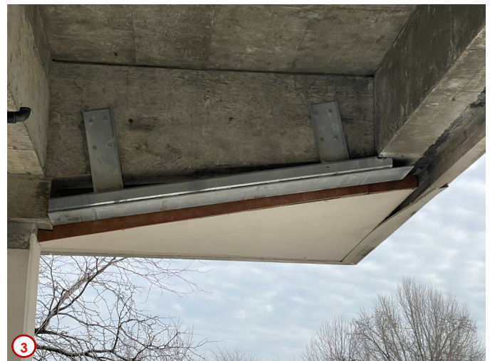
Photo #4 highlights the first few sections of the new curtain wall system for the addition at the northwest corner of the building. This area will house three huddle rooms as part of the new library layout. When completed the majority of the Library (other than the entry off of the new main corridor) will have views of the Little Pond which will help add to the interior environment for the building occupants.
