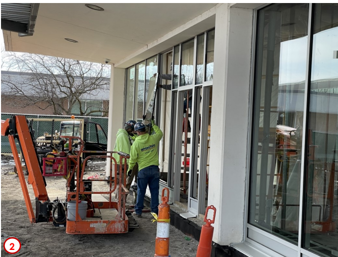
Photo #3 highlights the new structural steel that was installed at the edge of the existing soffit that will help support the new curtain wall system for the southeast addition.
