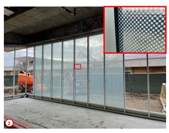
Photo #3 was taken later in the week and shows all of the glazing panels installed for the northwest addition. Now the contractors will focus on replacing and/or repairing the soffit adjacent to the additions to help weather-proof the envelop of the building. This addition will house huddle rooms for use by staff and students in the Library.
