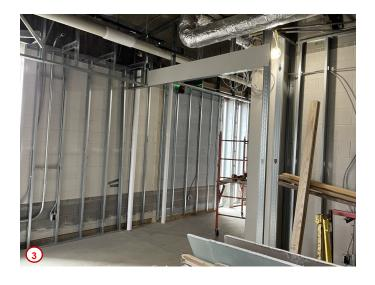
Photo #4 shows the Commons Area at the top of the western stair tower on the second floor and the last few sheets of wallboard being installed over the new framing and furring. Also happening in this area immediately around the perimeter of the stairs will be the framing for enclosure for the fire shutters.
