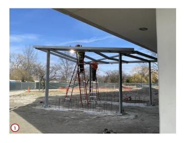
Photo #1 highlights the beginnings of the erection of the structural framing system for the new entrance canopy on the west side of the building. Here you can see the contractors welding some of the smaller cross members to each other to solidify the integrity of the entire structure.
