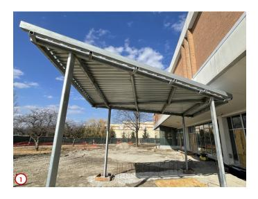
Photo #1 highlights the progress of the work needed to complete the new western entrance canopy. The structural steel for both canopies is now in place, and therefore the contractors can begin the process of installing the framing which will then lead to the finishes being installed.
