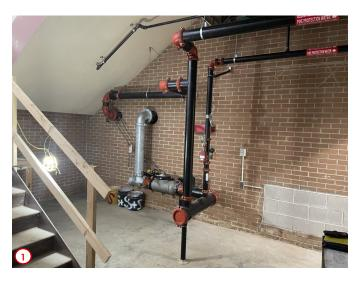
Photo #1 shows the progress of the installation of the new fire riser in basement near the west stair tower. Once completed the fire-rated partition that will help separate the new room in which this unit will reside will start being constructed.
