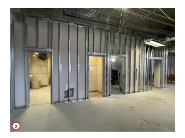
Photo #4 shows one of the many contractors at work on the first floor installing new light-gauge metal framing. Here the worker is trimming some newly installed metal studs that will provide the framework for the future bulkhead in the southeast addition that will provide a transition point for the suspended ceiling grid and the open ceiling that is part of the design aesthetics in the new computer lab and classroom in this area.
