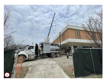
Photo #1 features the vacuum truck that was used to remove the existing stone ballast from the roof. In the background you can see the crane that has been set up to convey the new roof materials and needed installation equipment.
