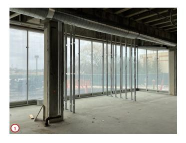
Photo #1 shows the progress of the installation of the rough framing in the northwest addition on the first floor. Here you can see the partition walls that will separate the future huddle rooms off of the Library being constructed.
