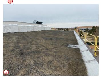
Photo #3 was taken on the upper portion of the roof and shows one set of the roof-mounted gooseneck mechanical louvers. Although these louvers were installed as part of the campus-wide geothermal HVAC system project the existing curb that they sit needed to altered and reflashed to work with the new roofing system.
