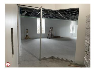
refurbished as part of the overall project. Here you can see the new suspended ceiling grid system now in place and ready for the electricians to install the new LED light fixtures.
