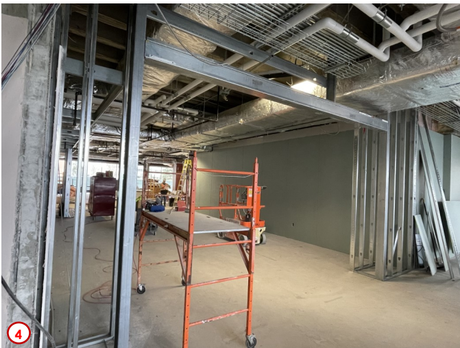
Photo #3 shows some of the carpenters installing the new gypsum board over the wall between the new classroom and the main corridor near the southeast addition. In the back you can see the voids between the metal studs have been filled with a fiberglass batt insulation to help cut down on noise transmission from the corridor into the classroom.
