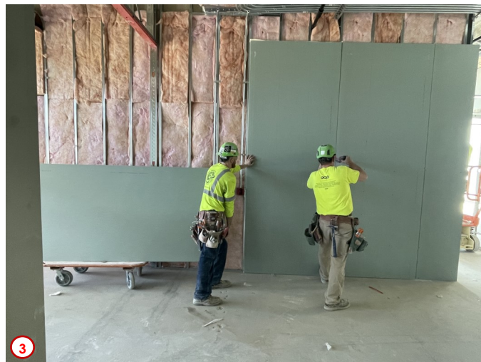
Photo #4 highlights the progress of the work needed to complete the rough framing for the entry into the new library area. The framing shown will help support the future overhead coiling gate which will help close off the library when not in use. This gate is similar to those you see at stores in a shopping mall. Unlike prior to the renovations this will allow the library to operate on different hours than that of the rest of building.
