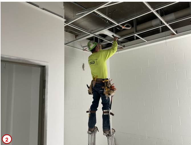
Photo #3 highlights more of the installation of some of the in-ceiling infrastructure. Featured in this photo is one of literally hundreds of diffusers that will help deliver conditioned air into interior of the building. You can also see the flexible duct connects to the trunk lines terminating into the top of this diffuser.
