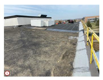
Photo #1 was taken along the east side of the lower portion of the roof. Here you can see an example of how the roofing contractors have been working in smaller sections. This way they can get the work accomplished even with the extra rainy weather we have been experiencing lately, and by doing this they are able to keep the interior of the building dry.
