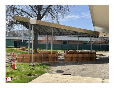
Photo #1 highlights the progress of the work on the new east entrance canopy. Here you can see more of the rough framing has been completed, and the formwork is in so that the concrete for the associated seating walls can be placed. This same process has been started for the new canopy on the west side of the building as well.
