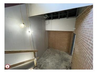
Photo #1 shows the beginning stages of the elevator replacement. Here the contractors are installing the sliding doors for the entry at the basement landing. The new machinery for the elevator was also replaced this week. In the next week the new cab will be assembled in place, and the remaining infrastructure installed as well.
