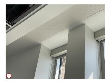
Photo #1 was taken in the staff lounge in the H/SS Division Office Suite looking at one of the grouping of windows. This photo features two new recently installed items the first being the new shades for the windows, and the radiant heat panels. The radiant heat panels are set into the soffit between the existing exterior wall and the new bulkhead, and help supplement for any heat loss caused by the windows.
