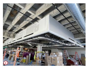
Photo #3 features one of the many new supplemental heating units now installed on the first floor. The unit featured in this photo is located at first floor landing in the east stair tower, and helps maintain the proper temperatures in this area due to any heat loss caused by the building occupants entering or exiting the building.
