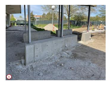
Photo #1 was taken outside at the new east entrance canopy. In the background one can see the landscaping work needed happening to install the new sidewalk that will connect the new east entrance to the central mall of campus for enhanced pedestrian traffic. In the foreground you can see that the concrete for the seating walls was placed this past week and await finishing.
