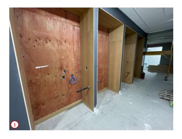
Photo #1 was taken in the north corridor near an area where some new student seating areas are being installed. This seating will feature single occupant restaurant-style booths that will feature lighted table tops to allow students to study or work on assignments.
