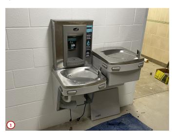
Photo #1 features one of the several new electric water coolers that are being installed throughout the building. Unlike the old units these are both ADA compliant and feature a bottle filling station which is a new standard that is being implemented campus-wide.
