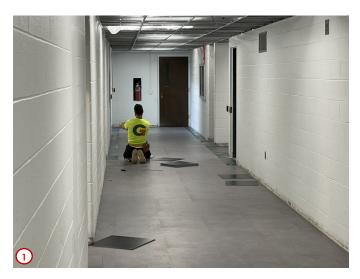
Photo #1 shows the flooring layers installing the LVT (luxury vinyl tile) in the basement corridors. Some of the main features we like about LVT over VCT (vinyl composition tile) is that it doesn't have to be stripped and waxed every year, and the color runs all the way through so scratches aren't as apparent. Therefore they are more robust and require less maintenance and therefore have a lower TCO (total cost of ownership).
