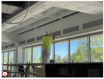
Photo #3 features the work that was happening near the new west entrance on the first floor. Here you can see the contractors installing the wallboard for the ceiling in the student commons area. Right next to that you can see the interior vestibule entry being installed at the same time.
