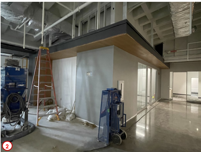
Photo #3 is similar to Photo #2 in that highlights more of the final finishes now installed. Here the entry into the new classroom on the west side of the second floor is nearly complete. The only remaining items are some finish trim and the application of the privacy film that will be installed on the glazing.
