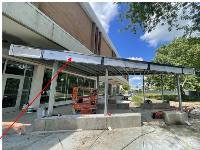
The top-right photo highlights the progress of the finishing of the new east entrance canopy. Here the new fascia cladding is being installed around the perimeter of the structure.
