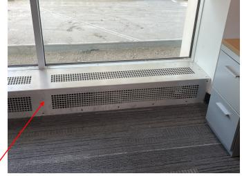
The top-right photo shows one of the new radiant fin tube covers was recently installed and that is typical for the perimeter of the first floor.
