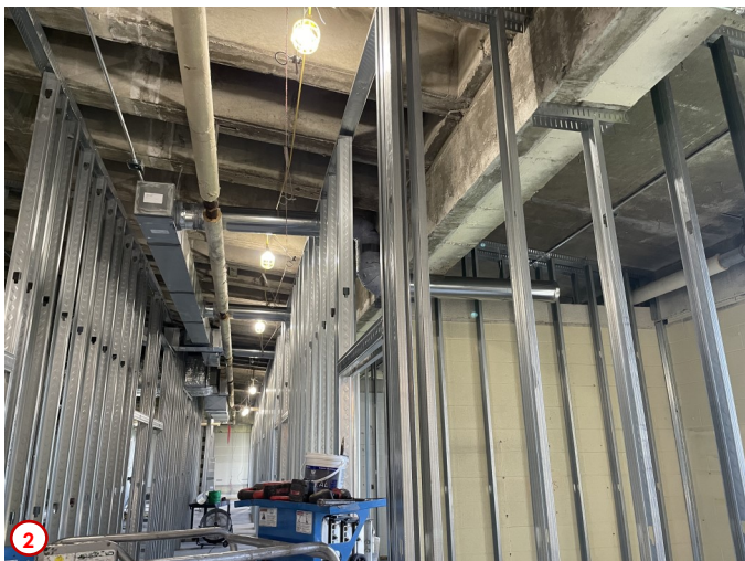
Photo #3 shows some of the rough framing going in for the future classroom that will occupy part of the space that formerly housed the LAL/ Disability Services and the Writing Center.
