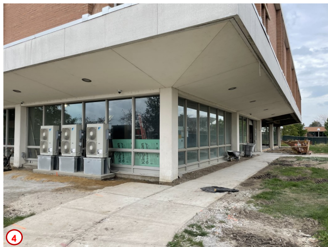
Photo #3 was taken in the same area as Photos #1 and #2 and shows more of the completed backfilling and site prep finished. This area will be where the future main west entrance to the building will be located and the associated canopy.
