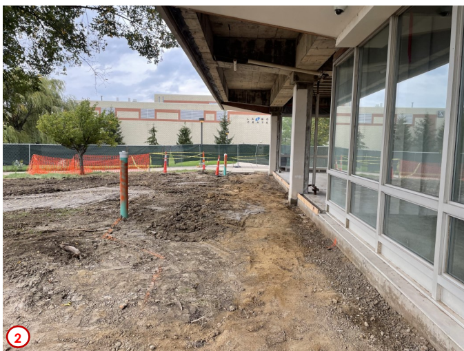
Photo #3 was taken in the same area as Photos #1 and #2 and shows more of the completed backfilling and site prep finished. This area will be where the future main west entrance to the building will be located and the associated canopy.
