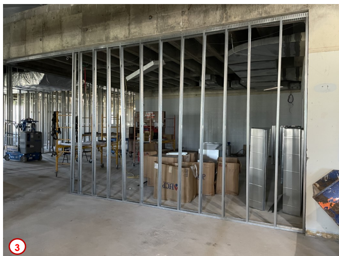
Photo #4 was taken along the west wall of the second floor near the west stairs and shows the very beginnings of the installation of the hydronic piping that will feed hot water to radiant panels that will line west wall and installed in the ceiling grid. These ceiling mount panels will replace the old units that used to line the base of the wall. The purpose of these panels is to help make up for heating or cooling loss from all the fenestration in the wall. This same scenario is happening in multiple places around the perimeter of the second floor.
