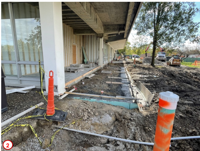
Photo #3 shows one of the contractors placing some concrete in an area where there is a depression from the old curtain wall system but needed to be built up so that it can bridge the gap between the existing and future floor slabs in this area.
