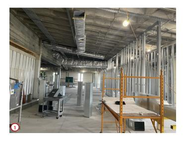
Photo #1 was taken in the area of the future H/SS Division Office Suite looking west. Along the right side you can see the stud walls forming that will be the faculty offices. On the left side you can see furring being applied to the existing masonry wall so that new wallboard can be installed. Then at the top you can see more of the existing ductwork has been insulated.
