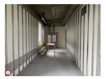
Photo #3 is a close-up detailed view of some of the new metal stud framing that will eventually form the faculty offices in the H/SS Division Office Suite.
