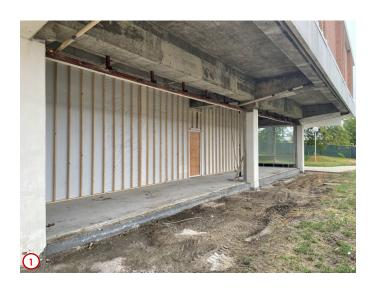
Photo #1 shows the now completed demolition of the old curtain wall system along the southeast portion of the first floor. In the next few weeks this area will be excavated so that the waterproofing system can be installed on exterior face of the basement wall. Once that is one the foundations for the addition in this area can be installed.
