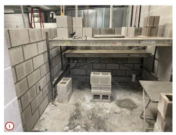
Photo #1 highlights the progress of the construction of the new janitorial closet in the basement of the CLRC. Again, the concrete for the floor slab has been placed and now the concrete block walls are being laid to fully enclose the space. You can see underneath the scaffolding the rough-ins for the future mop sink and oil separator along the east wall.
