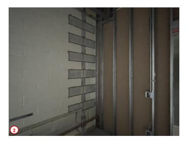
Photo #3 highlights the progress of the framing being done for the future single occupant study booths being constructed in the new north corridor between the classrooms and the H/SS Division Office Suite.
