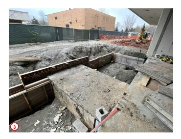
Photo #4 is another shot the formwork for the southeast addition on the first floor, but offers another perspective and provides a better idea of the size of this future space. The southeast addition is much larger than that which has already been started at the northwest corner of the building. This addition will house a classroom and computer lab when eventually completed.
