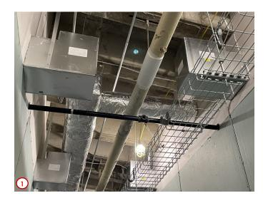
Photo #1 shows the progress of the installation of the fire sprinkler system on the second floor. Featured in this photo is a branch line running through the corridor in the H/SS Office Suite. The empty threaded connection will receive a down pipe that will terminate at one of the hundreds of sprinkler heads that will be eventually installed.
