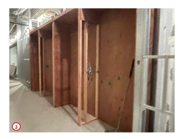
Photo #4 shows the progress of the installation of additional wallboard and framing in the east corridor. This corridor is existing and is receiving a wallboard finish on metal furring channels. This new finish will not only be more attractive than the existing masonry walls, but will also help with acoustical legacy items and will hopefully cut down dramatically on the echoes that used to plague this area.
