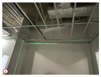
Photo #3 shows more building insulation having been installed in the stud spaces in the new wall framing. With these walls being interior the insulation isn't for heating and cooling reasons, but rather to help provide acoustical separation for the classrooms from the adjacent corridors.
