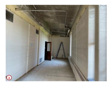
Photo #4 was taken in the south corridor looking east. Similar to the rest of the second floor all of the old finishes have been removed along with the required abatement completed. Now the contractors are focusing on disconnecting all of the existing HVAC and electrical connections in order to allow for wall demolition and eventually new construction as much of the second floor will be rearranged to better fit the new spaces being programmed in that area.
