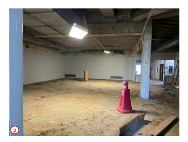
Photo #3 highlights the progress of the demolition work happening in the existing offices. This area used to divided up for the Dean of H/SS Division and the Administrative Assistant. You can see that similar to the adjacent classrooms all existing finishes have been removed.
