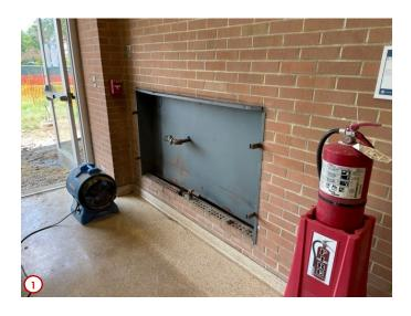
Photo #1 is of the first floor landing in the west stair well. Here one can see that the existing supplemental unit heater has been removed so that the wall it use to reside in can be removed per the new plans developed by the architect for the project.
