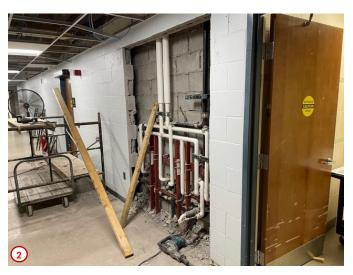
Photo #3 shows the corner of the existing mechanical room in the basement where the new janitor's closet will be constructed. Using GPR (ground penetrating radar) the contractor has noted the location of all the existing utilities and infrastructure located under the slab prior to the removal of the existing concrete floor slab and associated excavation.
