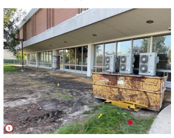
Photo #1 shows the site preparation that has been done already to prepare the installation of the new entry system on the west side of the first floor, as well the erection of the new entrance canopy and land-scaping walls. This is part of the effort to change the 'back door' on the west side of the building into a new 'front door' off of Lot 7.
