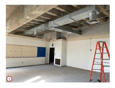
Photo #1 was taken in one of the existing classrooms. In all the classrooms that are being updated they will receive new finishes (ceiling and LED lighting, flooring, furniture, and A/V technology. All of the entryways will also be updated to meet with new accessibility code auidelines.
