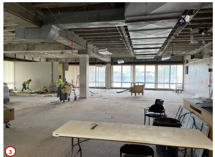
Photo #2 shows the progress of demolition that is happening near the area of the elevator. This work is very symbolic as these walls are the last remaining barriers that stand and soon will be gone so that this building will finally be barrier free and therefore ADA compliant. After all of the walls surrounding the existing elevator shaft are gone the contractors can start erecting the new framing that will become the new first floor corridor that will connect the new east and west entrances as well as allow free access to the vertical circulation routes.
