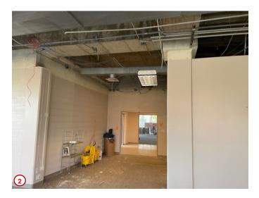
Photo #3 show more of the progress in the old Library space. In this photo one can see that the old HVAC ductwork supplying this area is being removed. Soon the remainder of the walls and floor finishes in this portion of the building will be removed as well to permit the contractors to erect the framing per the proposed layout. This particular area will be the location of the new office suite and partially the entrance gallery into the library.
