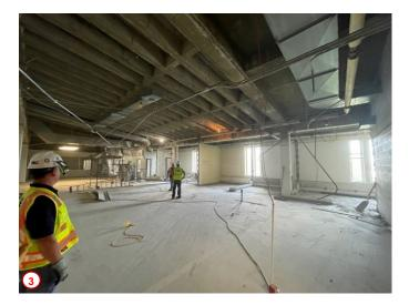
Photo #4 was also taken later in the week and shows the walls gone between the corner classroom and the old LAL space. Again, new framing for the H/SS Office Suite will be installed in this area as well as the necessary infrastructure for the new adjacent corridor. The contractor will be focused on the west side of the floor next week as far as demolition goes.
