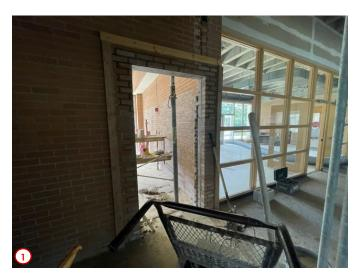
Photo #1 highlights the progress of the work at the first floor landing of the eastern stairwell. Both of the old double door openings have been filled in with cmu and existing brick, and then the new single door opening has been cut in and salvaged brick is being used to finish out the opening so the new door frame can be installed. This change was necessary to facilitate the new Library Staff Office Suite which will be partially located where the old main entrance to the space was located.
