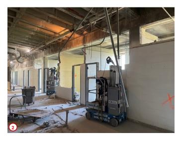
Photo #3 was taken later in the week after the previous two photos and shows the fact that all the walls in that area were removed and the debris cleaned up and properly disposed of. Soon new framing will be installed per the architect's plans.
