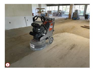
Photo #1 shows the progress of the removal of the mastic that was used to adhere the carpeting once in the Library to the floor slab. It was necessary to remove this to allow for the new wall framing, and so the new flooring to be installed in this area will be properly adhered to the slab and warranted by the manufacturer.
