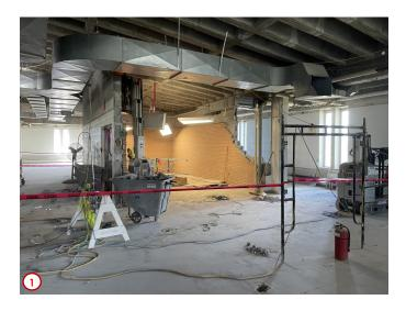
Photo #1 shows the progress of the start of the last major demolition work in the CLRC, and that is the removal of 3 of the 4 walls of the west stair on the first and second floors. These walls will be replaced by a retractable fire curtain that will deploy in case of a fire emergency. The removal of these walls will allow the creation of the open floor plan that was desired and to aid the infiltration of more natural light into the building interior.
