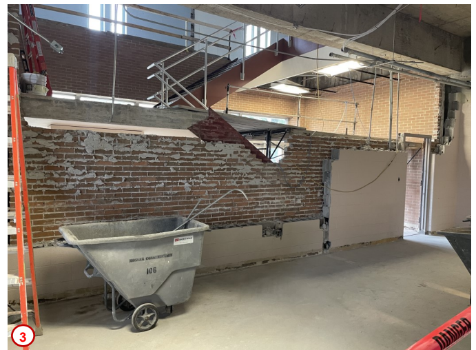
Photo #4 shows some additional infilling of the existing concrete block wall that used to separate the old janitor's closet and staff lounge. The new block were tuck-pointed in and new framing and finishes can be installed in accordance with the architect's plans for the new layout of spaces in this area.
