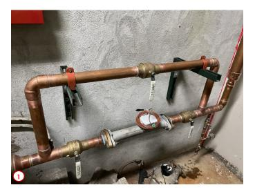
Photo #1 was taken in the northeast storage room under the eastern stainwell, and highlights the new domestic water feed and meter/valve for the building. The old domestic water feed was tied into the old fire riser that will be demoed as the new fire riser will located in the western portion of the building. The new valve (highlighted for your reference) has a new remote digital reader integrated into it which will allow for more accurate monitoring.
