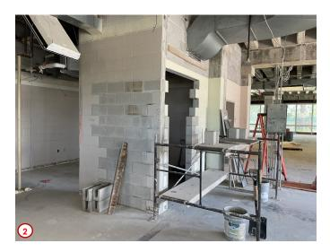
Photo #3 was taken near the old entry into the area that was the Quiet Study Area for the Library. As you can see the old entry is now blocked off by a new concrete block wall. This wall was necessary in order to create the proper flow in and out of the revamped and resized Library.
