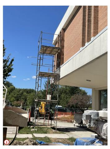
Photo #2 is an exterior shot on the south side of the building looking west. Here you can see scaffolding going up that will allow the contractors to convey building materials to the second floor through an existing window. This work was needed in preparation for the aforementioned elevator replacement that will hopefully start soon. Once the new elevator is in it will be kept offline for conveying materials and workers so as to help protect it from damage.
