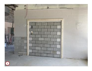
Photo #1 was taken in the area of the old Quite Study Area of the Library. The new concrete block shown filled in the opening where the old double doors leading into the receiving area used to be located. This wall when finished will help to serve as a barrier between the revamped receiving area and the new café/student lounge along the south side of the new main first floor corridor.
