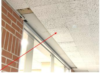
The top-right photo shows the installation of the new spline ceiling tiles that match the existing in the area.
