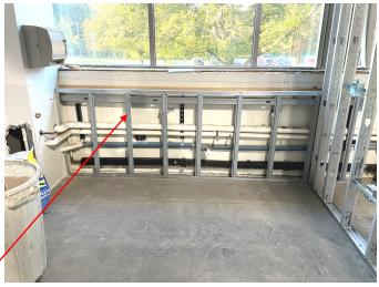
The top-right photo shows some of the new metal stud furring strips being installed on the south face of the future Student Government Room. This framing will help to conceal the existing plumbing in this area and provide a wall for some future cabinetry to be installed at a later time.
