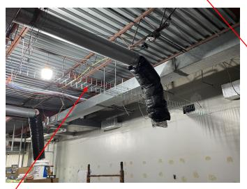
The bottom-left photo shows the remaining portion of the cable tray for this space now properly installed and ready to house future information systems communication lines. This cable tray connects across the corridor to the new set installed there and eventually terminates in the south IT Room.
